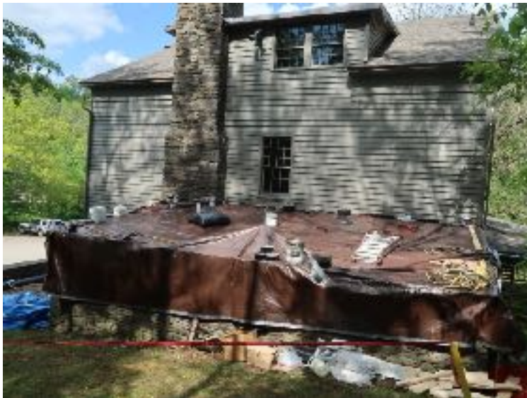
Figure 4. Work on the mill roof replacement.
